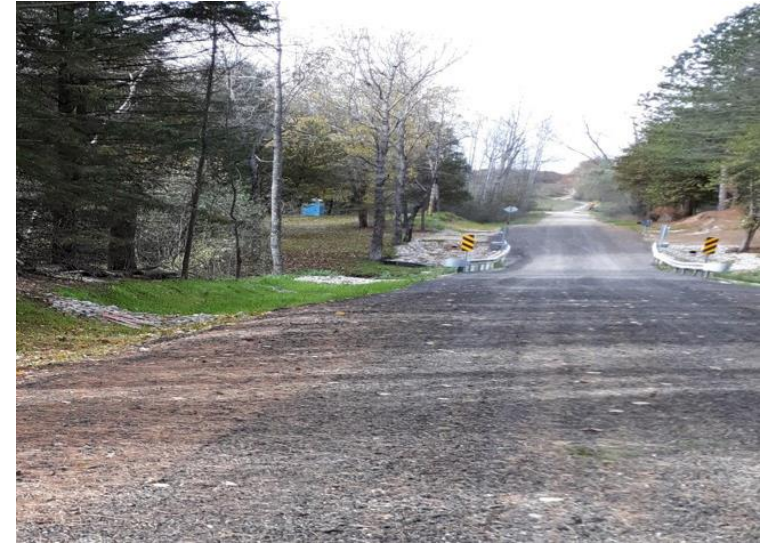
Stockwell Over Middle Branch Cedar River After Streambank Stabilization 2018, Hamilton Township
