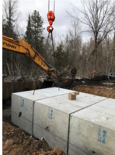
Athey Over Cranberry Creek During Culvert Replacement 2018, Hamilton Township
